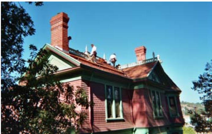
Roofers working on Hale House roof.
